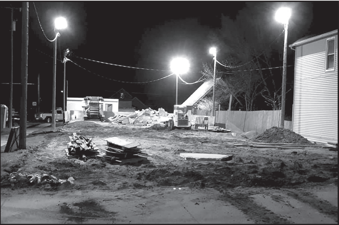
The machine (left) is owned by Kurt Gillund of Rite-Way Drainage. He will be using that machine sometime in May to crush the concrete slabs piled up next to it. This week the fencing around the rink went down Special Photo.
